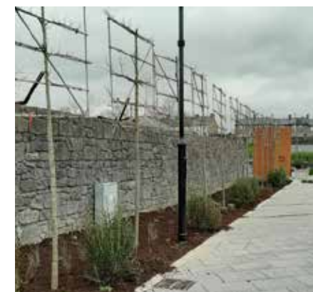
Limestone Mortar wall to North Circular Rd.
