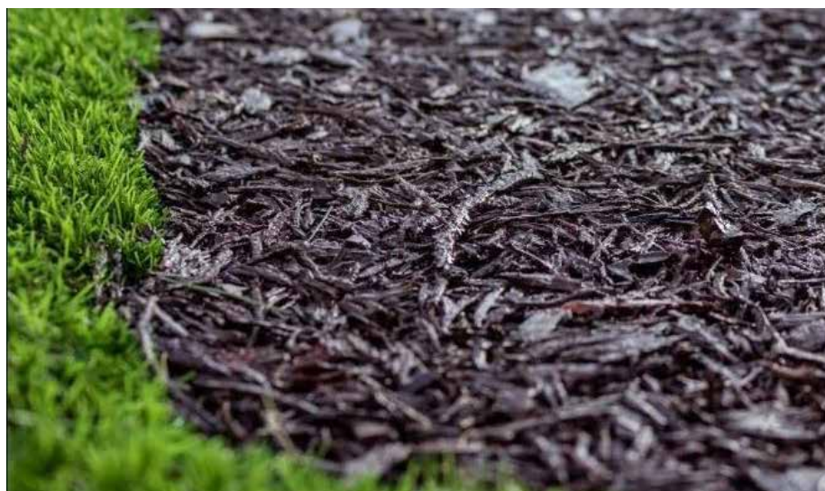
Resin bonded recycled rubber mulch safety surfacing for Older children's play, climbing and Fitness court in the Quarry
